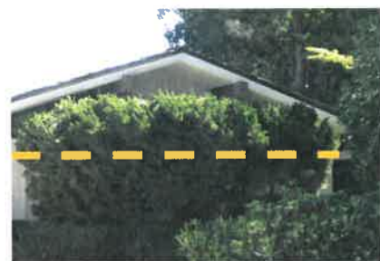
Shrubs should be less than one-half the height to the eave
