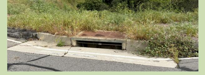
Road drains have been engineered and designed to take water from the streets to the natural drainage courses. Blocking a drain can overwhelm other downhill drains and cause damage.
